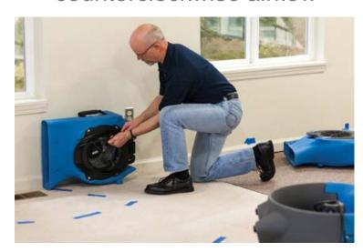
Wall & floor drying clockwise airflow
